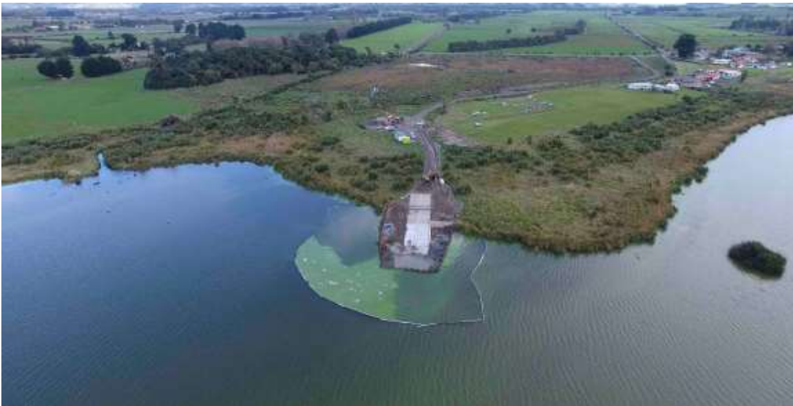
Figure 19: The Lake Horowhenua boat ramp prior to the removal of the sheet piling and sediment curtain. The current sediment trap and proposed wetland site can be seen in the background.
