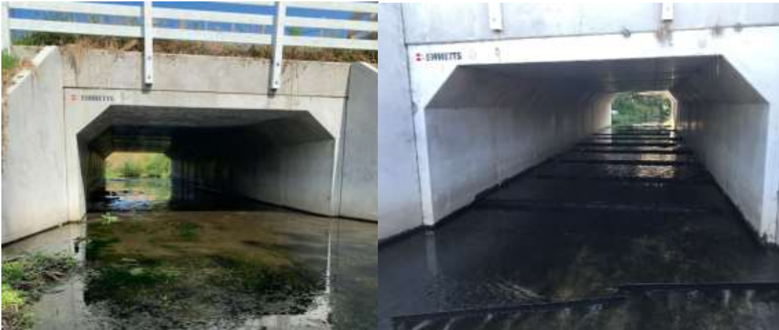
Figure 7: Left: Large box culvert located in the Awarua Stream, Whanganui, prior to remediation. Right: Remediated culvert with lengths of flexi-baffles and a fish ramp installed.
