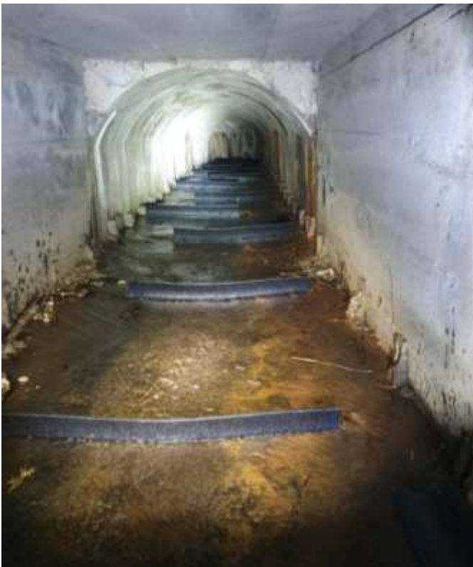
Figure 8: Culvert remediation, Purua Stream, Whanganui. Flexi-baffles were installed throughout this 195 metre culvert running under SH4 into the Whanganui River.
