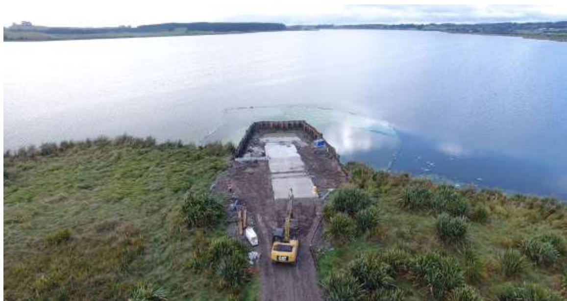
Figure 20 The Lake Horowhenua boat ramp prior to the removal of the sheet piling and sediment curtain.
