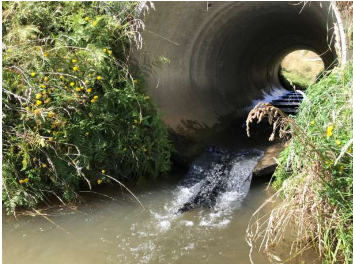
Figure 16: This culvert in the Waoku Stream catchment, a sub-catchment to the Koputaroa, had a small perch. This was remedied by placement of rubber matting and mussel rope.
