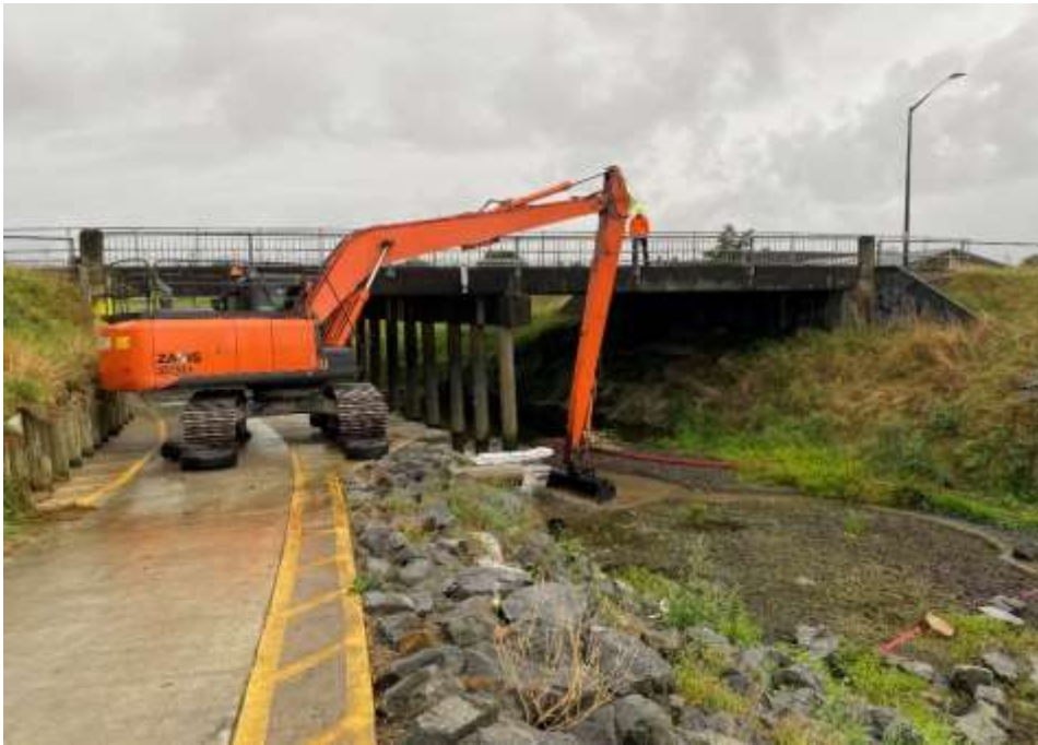
Figure 3 Long reach digger removing rooted alligator weed plants in gravel beach. (K.Hoggard)
